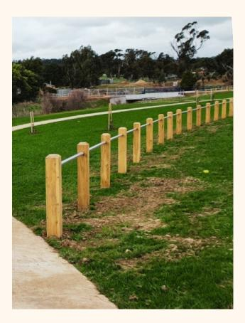
Ensuring the use of appropriate timber to withstand the weather and low maintenance is vital to their longevity. So too is the correct installation. Installation can be either using earth and cement slurry or in concrete footing. We have outlined the installation process for both options on the following pages.
